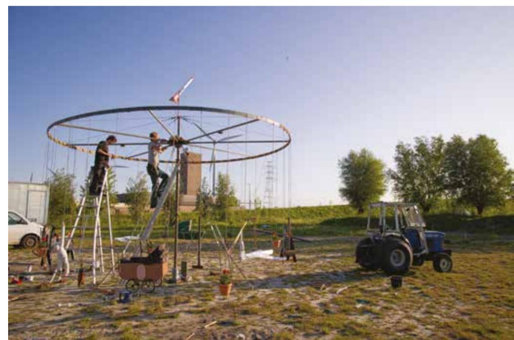
*"The hardest part was anchoring the tension cables that stabilised the axle. The merry-go-round was set in motion by a nicely coiled and greased steel cable of 50 meters long, which was pulled by a tractor that slowly drove away."*
